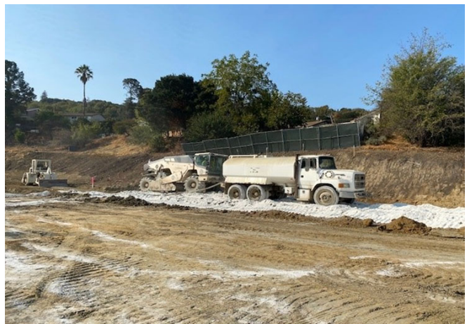
Begin lime treatment of subgrade
